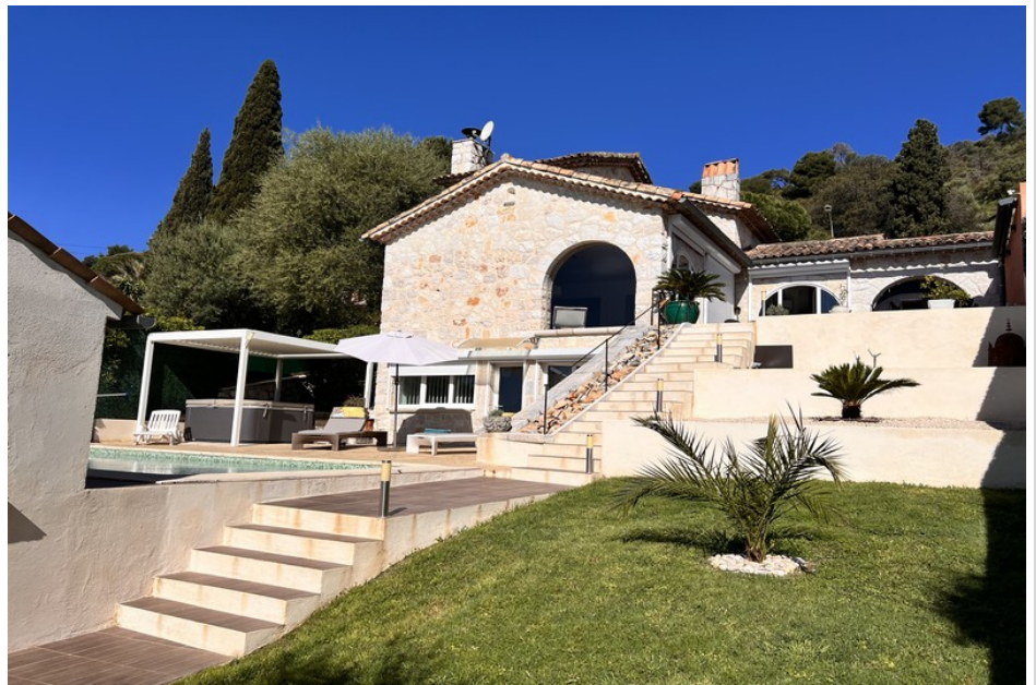
House 600 La Colle-sur-Loup
